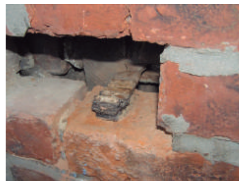
Connector cavity wall. Font http://www.repointing-brickwork.com/brickwork/wall-tie-replacement/
